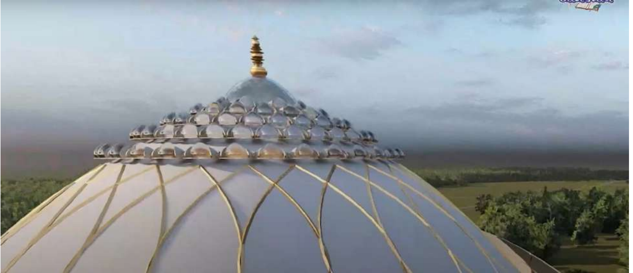
Resembling clear dew drops, the pinnacle of the lotus bud adorns glass skylights at 5 levels to filter in sun rays into the inner sanctum. Image source: Vastu World
